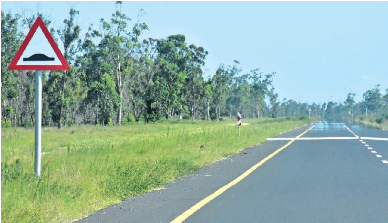
Figure 3. Placement of speed bumps and speed limit signs on the Maputo National Park road, as a measure to minimise possible collisions between vehicles and medium or large wild animals, which can result in serious road accidents and the deaths of both people and animals (Credit: Idnórcio Muchanga).
