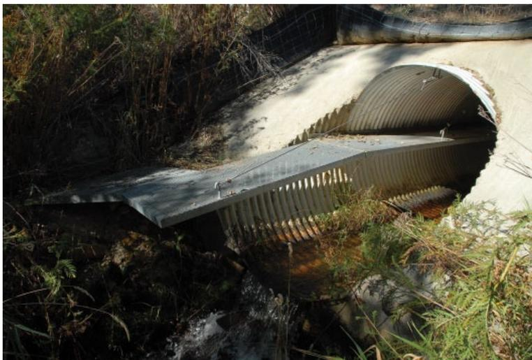
**Figure 35.7** Bolt-on wildlife shelf retrofitted to an existing drainage culvert for use by weasels. Source: Photograph by and reproduced with permission of Kerry Foresman, Critter-Crossing Technology L.L.C.
