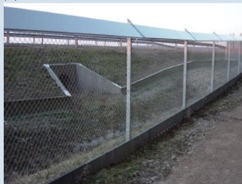
**Figure 35.10** (A) The European wildcat is identified by the circular black rings on its tail. (B) Fences for wildcats in Germany are 2 m high with mesh size of 5 cm<sup>2</sup>, a 50 cm-wide overhanging metal sheet and plastic board buried 30 cm deep. Source: (A) Photograph by and reproduced with permission of Heiko Müller-Stieß; and (B) Photograph by N. Klar.
