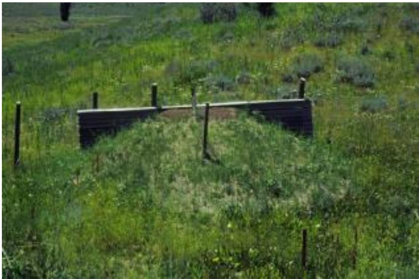
**FIGURE 2** Example earthen escape ramp (19).
